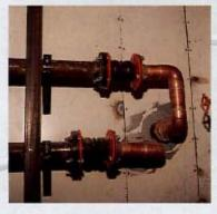
Even a very fragile copper pipeline with sweat fittings will survive at the equipment interface if proper flexible joints are used. This system was subjected to approximately 0.2gV and 0.2g9H, and showed no signs of failure because of the flexibility of the twin sphere rubber connectors. (Mason Twin Sphere Superflex shown. Current improved design is Mason Safeflex.)
