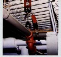
The clevis hanger in the center of the photograph full apart and the rear hanger clevis is sufficiently displaced to have bent the ceiling bolt. There are chatter marks on the pipe in the front clevis, all indicating that this system went into resonance even though the accelerations were only 0.15gV and 0.2gH. Proper sway bracing, axial restraint and upper limit stops could have prevented this damage,
