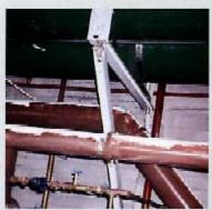
The swivel sway brace fittings at the ends of the angle iron brace eliminate welding, fitting and fabrication time. Solid sway braces can only be used on equipment that is not isolated. When equipment is isolated, bracing must be by cable or isolated devices to prevent transmission of vibration. (Mason 558)
