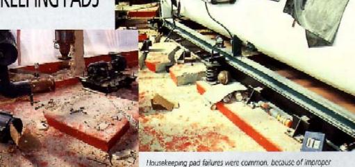
doweling or fastening to the structural floor, and inadequate or no reinforcement in the pad itself. These pads, as the pads on the cover, had both problems. Inadequate fastening allows the pads to lift, chatter and shift. Pour reinforcement allows breakage. When the pads
