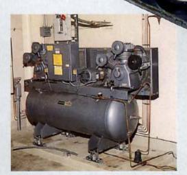
This is a simple isolation method for a horizontal tank mounted compressor (if the base legs are sturdy enough) without the use of a supplementary steel base. Mountings have built in seismic snubbers with ratings from OSHPD in the State of California. Not only these mountings, but similar designs were successful in every reviewed location. Forces were approximately 0.2gV and 9.25gH. (Mason SLRA Mountings)
