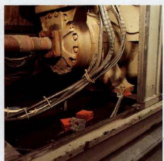
The cable system is an emergency measure to try to keep the compressor in place in anticipation of after shock. Forces were small at approximately 0.15gV and 0.2gH. Equipment with hard mounted internal components and external cushioned seismic isolation systems have a better chance of remaining operative.
