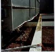
The independent rails rotated around their longitudinal axis, snapping anchor bolts and bending the cooling tower base. The problem could have been prevented by using a one piece structural base and double acting snubbers.
