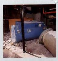
Water heaters have high centers of gravity and tend to turn over easily. The forces on this particular Installation were 0.15qV and 0.2gH, heaters should be bolted to the floor and strapped to the nearest wall or column.
